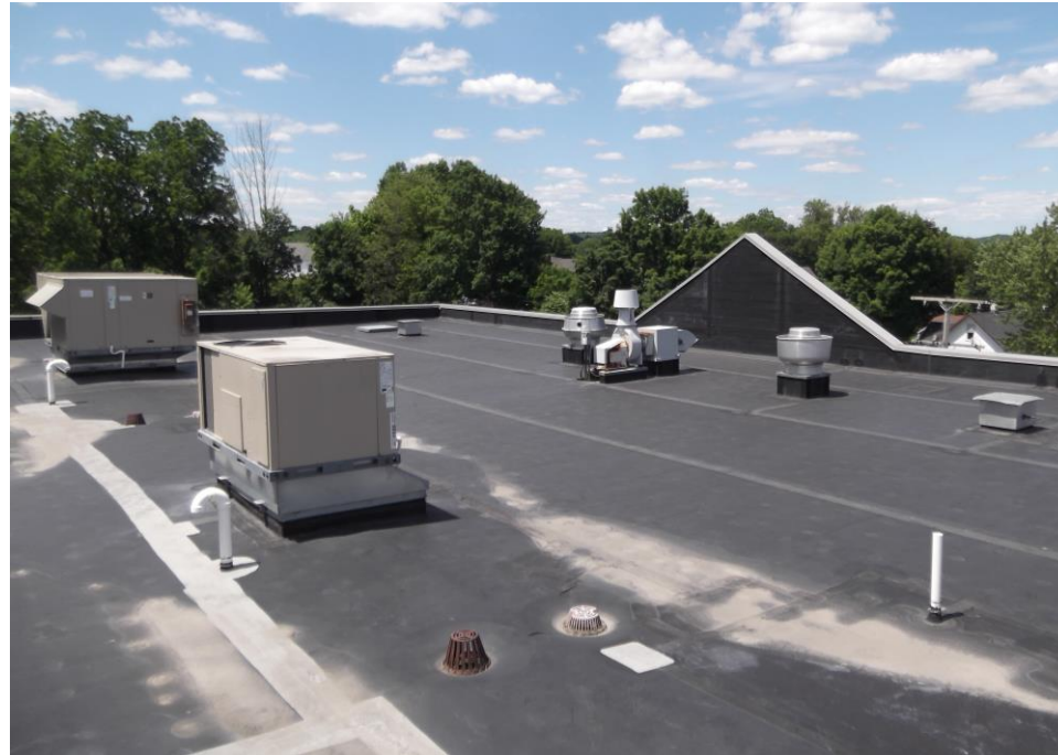
Rubber Roof New Addition
