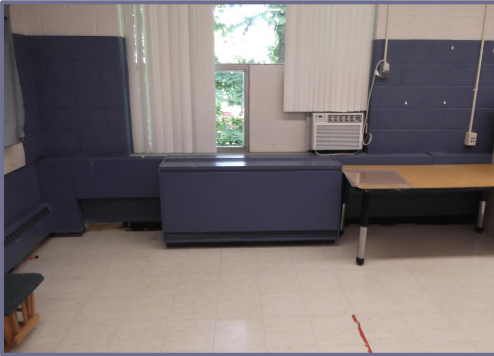
Unit Ventilator – Pic #1
